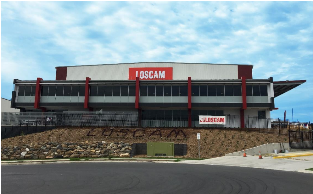
Loscam Sydney Erskine Park Depot, 54 Tyrone Place NSW 2759
